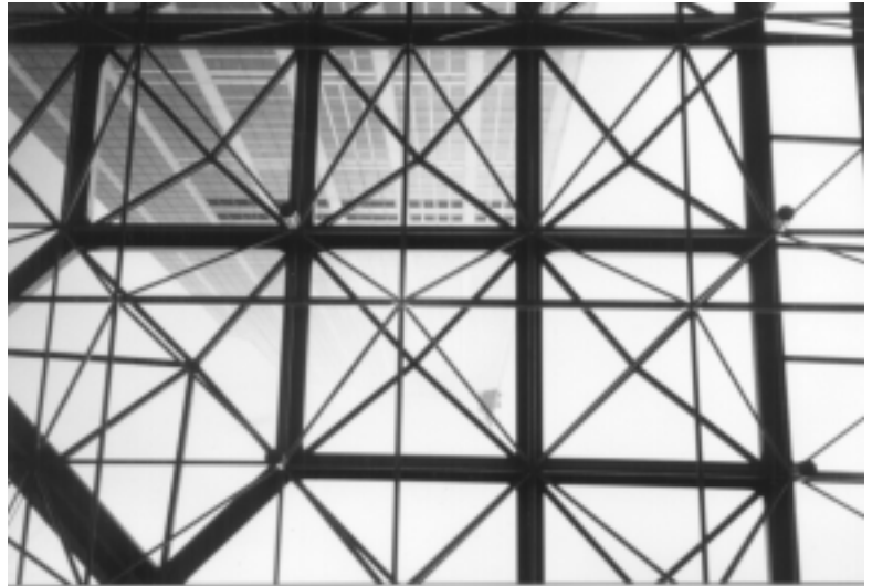
Figure 7.3. Scaffolding above Melbourne Central train station entrance.
