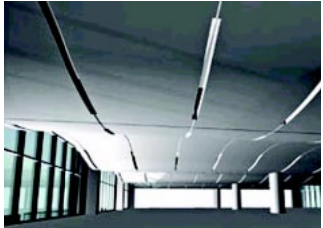
Overnight fresh air will cool the thermal mass of the unique wavy cement ceilings.
