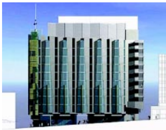
Southern facade showing three-storey-high shower towers facing Little Collins Street. The light-coloured southern façade where cool fresh air would be drawn in and down through the building.
